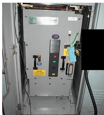
Before and After Installation of a New Cell Retrofit and Installation of Replacement PowlVac® Breaker
