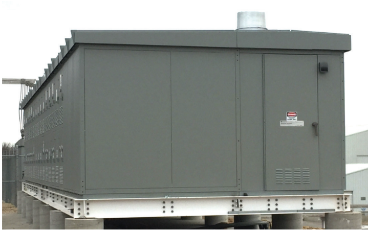
Typical Powell Power Control Aisle™ Installation with a structural steel skid mounted on concrete piers
