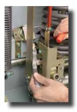
11. Slowly depress the trip coil armature using the manual charge handle.
