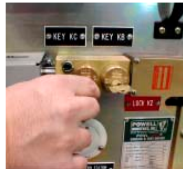
Figure 87. Transfer Key KC to Key Lock K2 and Rotate
