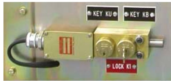
Figure 21. Key KB is Captive and Key KU is available
