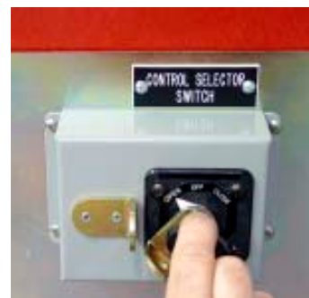
Figure 95. Move the Control Selector Switch to the OPEN Position
