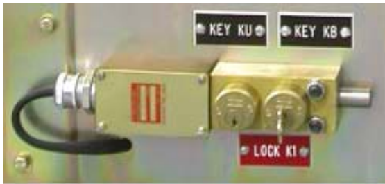
Figure 3. Key Lock K1 Interlock
