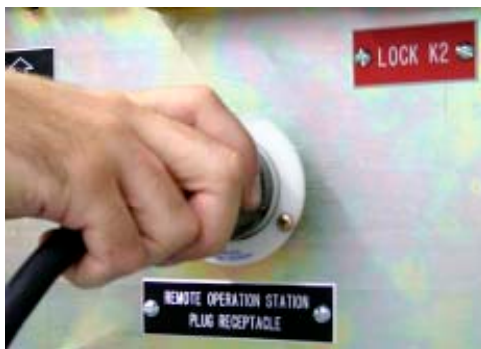
Figure 55. Connect the Umbilical Cord of the Remote Operating Station to the Ground and Test Device
