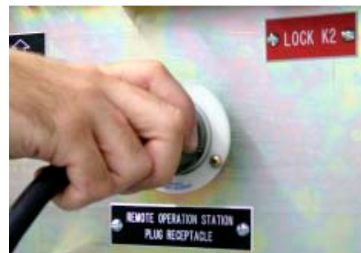
Figure 40. Connect the Remote Operating Station Cord to the Ground and Test Device and Rotate
