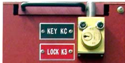
Figure 34. Insert Key KC in Key Lock K3 and Rotate
