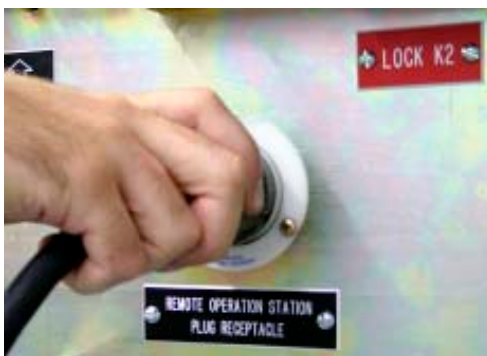
Figure 64. Connect the Umbilical Cord of the Remote Operating Station to the Ground and Test Device
