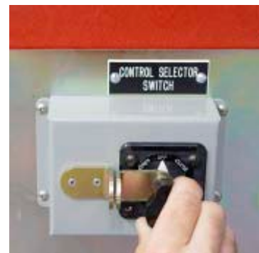
Figure 77. Verify that the Control Selector Switch is in the OFF position
