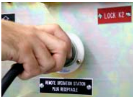
Figure 68. Disconnect the Remote Operating Station Umbilical Cord from the Ground and Test Device
