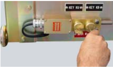
Figure 90. Insert key KB to Key Lock K1 and Rotate
