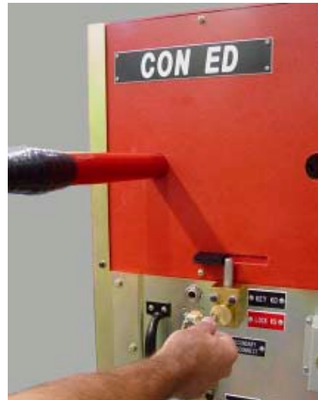
Figure 50. Install the Test Probes in the Test Ports
