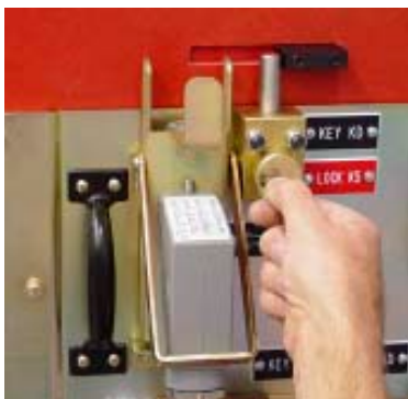
Figure 74. Rotate the Key KD to Unlock the Test Port Shutters
