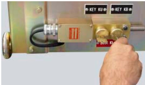
Figure 53. Transfer Key KB to Key Lock K1 and Rotate
