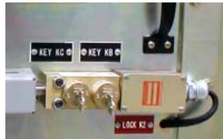
Figure 4. Key Lock K2 Interlock
