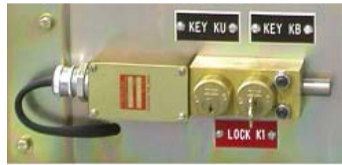
Figure 91. Key KB is Captive and Key KU is available
