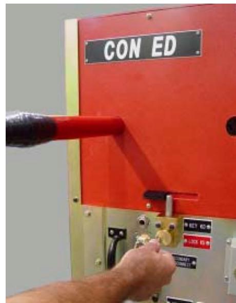
Figure 73. Remove the Test Probes from the Test Ports
