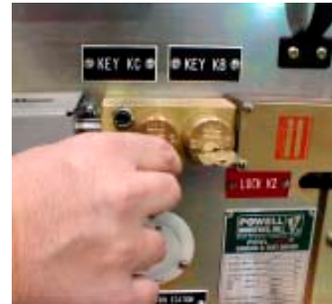
Figure 19. Transfer Key KC to Key Lock K2 and Rotate
