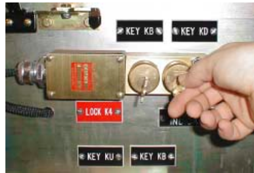
Figure 52. Transfer Key KD to Key Lock K4 and Rotate
