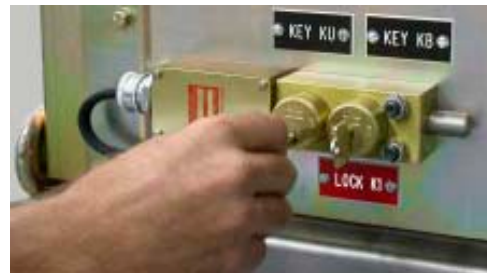
Figure 89. Remove Key KU from Key Lock K1
