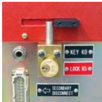
Figure 7. Key Lock K5 Interlock
