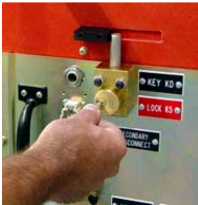
Figure 51. Rotate Key KD to Lock the Test Probes
