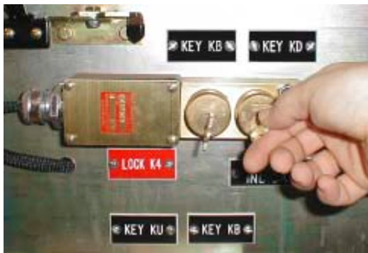
Figure 47. Transfer Key KB to Key Lock K4 and Rotate Key KD
