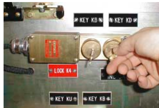
Figure 75. Transfer the Key KD to Key Lock K4 and Rotate
