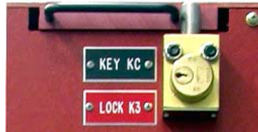
Figure 103. Push the Racking Access Interlock Handle in Fully
