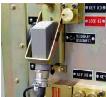
Figure 94. Connect the Compartment Secondary Disconnect to the Receptacle on the Ground and Test Device
