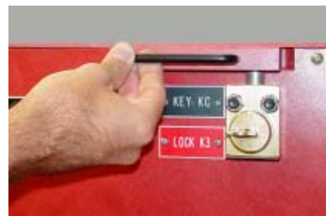
Figure 101. Transfer Key KC to Key Lock K3 and Rotate
