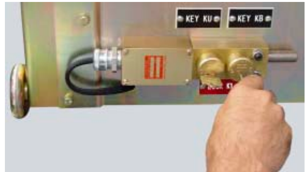
Figure 61. Transfer Key KB to Key Lock K1 and Rotate
