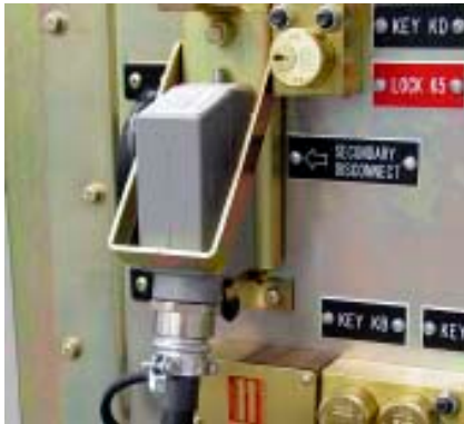
Figure 24. Connect the Compartment Secondary Disconnect
