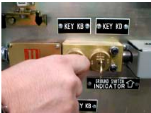
Figure 70. Transfer Key KB to Key Lock K4
