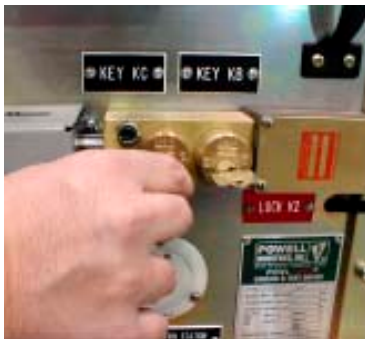
Figure 104. Transfer Key KC to Key Lock K2 and Rotate
