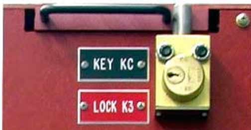
Figure 5. Key Lock K3 Interlock
