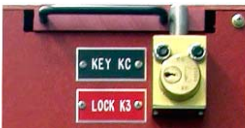
Figure 16. Insert Key KC in Key Lock K3 and Rotate
