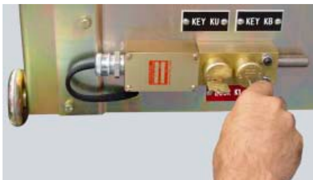
Figure 76. Transfer Key KB to Key Lock K1 and Rotate
