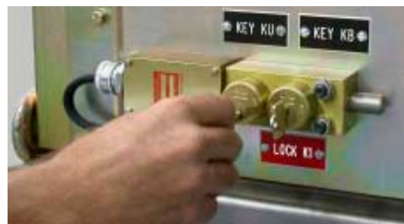
Figure 69. Rotate Key KU in Key Lock K1 Electrically Locking the Ground and Test Device CLOSED
