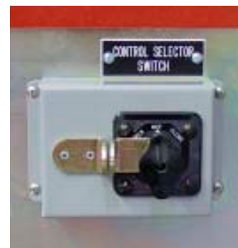
Figure 8. Control Selector Switch
