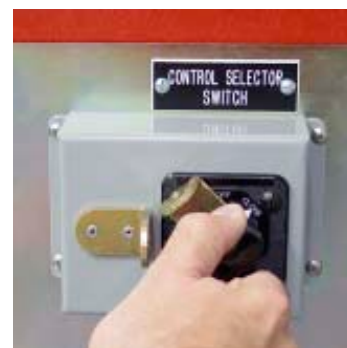
Figure 65. Move the Control Selector Switch to the CLOSE Position
