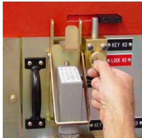
Figure 48. Transfer Key KD to Key Lock K5 and Rotate
