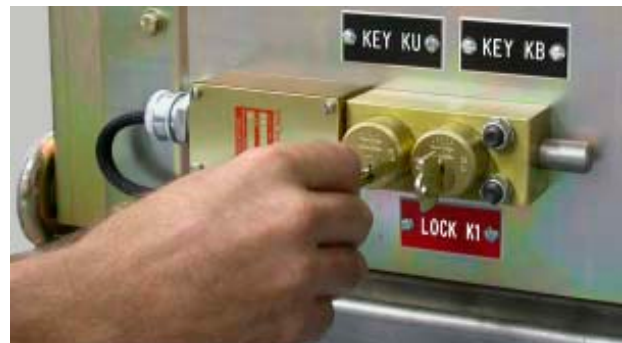
Figure 99. Rotate the Key KU in Key Lock K1 Key KU is captive and KB is available
