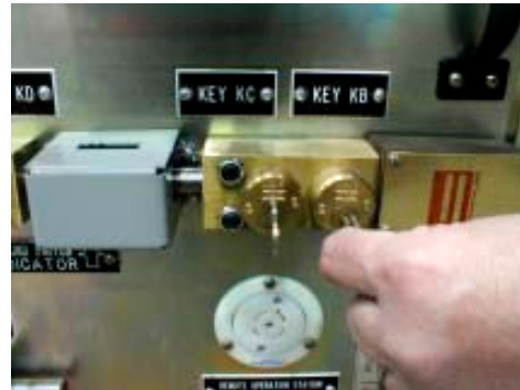
Figure 85. Transfer Key KB to Key Lock K2 and Rotate
