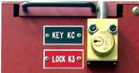
Figure 18. Rotate Key KC to Lock the Ground and Test device in the CONNECT position
