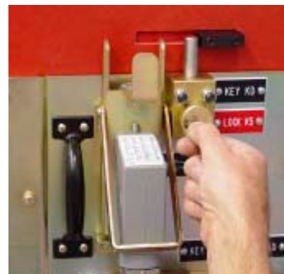
Figure 71. Transfer Key KD to Key Lock K5
