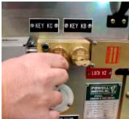
Figure 37. Transfer Key KC to Key Lock K2 and Rotate
