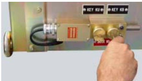
Figure 88. Transfer Key KB to Key Lock K1 and Rotate
