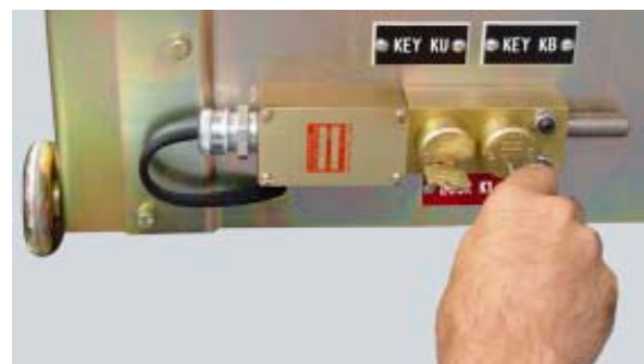
Figure 46. Rotate Key KB in Key Lock K1
