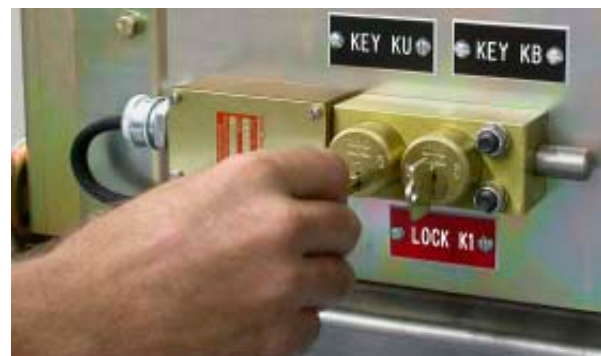
Figure 83. Rotate Key KU in Key Lock K1
