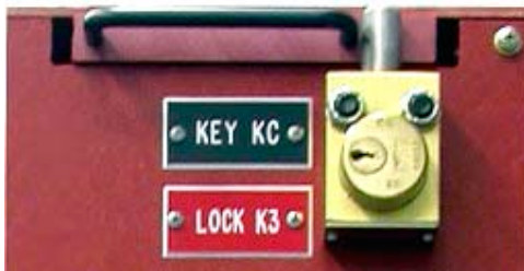
Figure 86. Transfer Key KC to Key Lock K3 and Rotate
