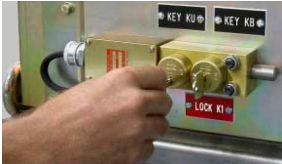
Figure 29. Rotate Key KU in Key Lock K1
