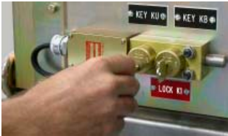
Figure 12. Insert Key KU into Key Lock K1 and Rotate Key KB
