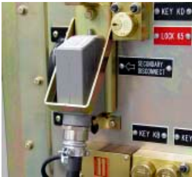
Figure 84. Disconnect the Compartment Secondary Disconnects from the Ground and Test Device
