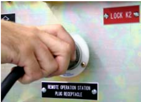
Figure 98. Disconnect the Remote Operating Station Umbilical Cord from the Ground and Test Device
