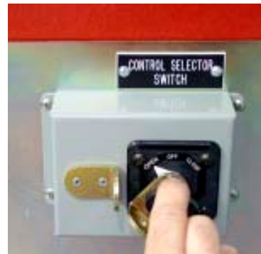
Figure 79. Move the Control Selector Switch to the OPEN position
