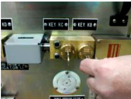
Figure 14. Insert Key KB in Key Lock K2 and rotate Key KC
