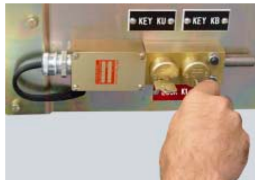
Figure 60. Rotate Key KU in Key Lock K1 Electrically Locking the Ground and Test Device OPEN
