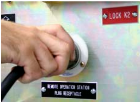
Figure 78. Connect the Umbilical Cord of the Remote Operating Station to the Ground and Test Device
