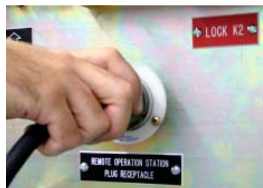
Figure 23. Connect the Remote Operating Station Cord to the Ground and Test Device and Rotate to Lock
