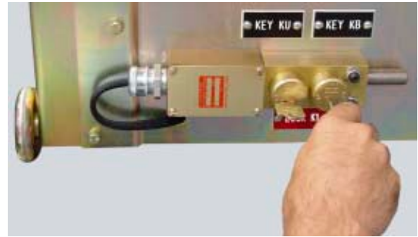
Figure 30. Remove Key KB from Key Lock K1
