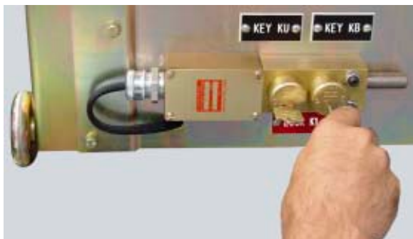
Figure 20. Transfer Key KB to Key Lock K1 and Rotate
