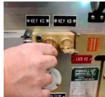
Figure 15. Rotate Key KC
