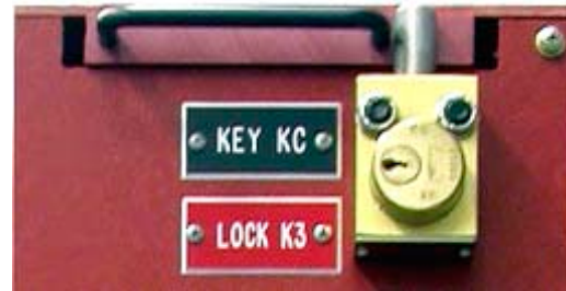
Figure 36. Rotate Key KC to Lock the Ground and Test Device in the CONNECT position
