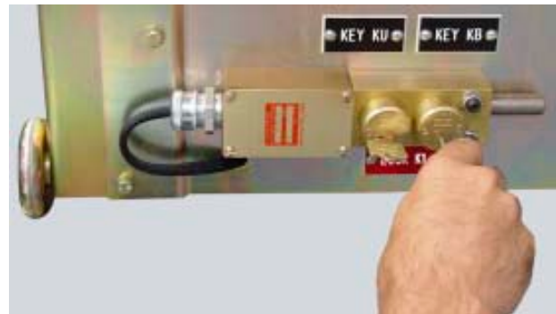
Figure 38. Transfer Key KB to Key Lock K1 and Rotate
