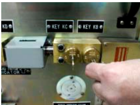
Figure 100. Insert Key KB into Key Lock K2 and Rotate
