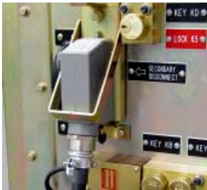
Figure 41. Connect the Compartment Secondary Disconnect to the Receptacle
