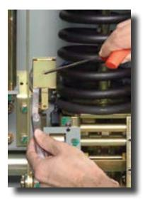
12. Slowly depress the trip coil armature using the manual charge handle.
