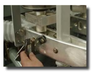
v. Lubricate the pin with a liberal coat of A - Grease. Insert the pin through both the bell cranks and the operating yoke, and place a new X-washer in the groove of the pin. Tighten the X-washer by squeezing the two open ends together with pliers. It may be necessary to align the operating yoke and bell crank holes to allow pin insertion. This can be accomplished by applying a downward force to the lower contact block just sufficient to overcome the force of the vacuum.
