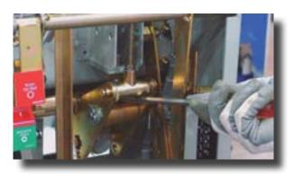
e. If present, loosen the set screw holding the operating yoke to the operating pin. Remove the X-washer from one end of the vacuum interrupter operating pin and remove the pin (Figure 29). The X-washer can be opened by squeezing the two projecting tabs with pliers. Discard the X-washer after removal.
